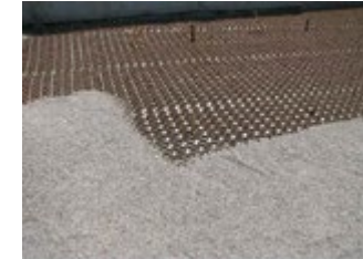
GRAVELPAVE2 DURING INSTALLATION
