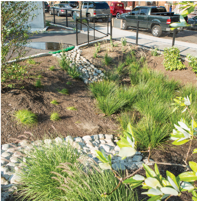
Green infrastructure like trees, rain gardens, and bioswales prevents flooding on schoolyards, making them available for play throughout the year. Those features also capture stormwater during rain events, improving water quality in local rivers, streams, and bays. Photo: Nick Benson Photography (top); Photo: Jenna Stamm (bottom)
