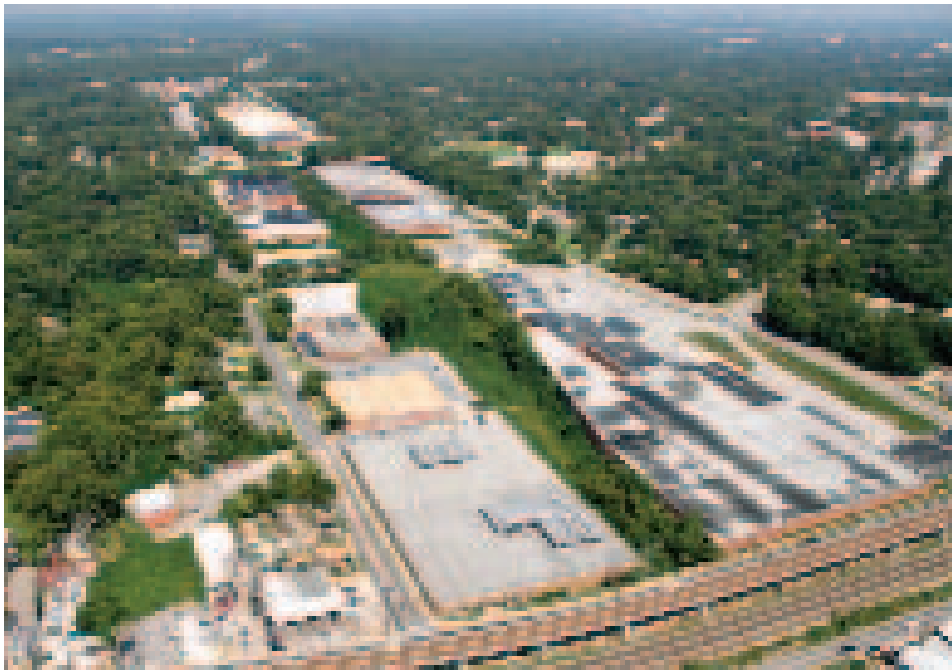
Left: Murphy Crossing looking northwest
