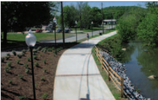
Above: Before and after PATH trail conversion along a creek
