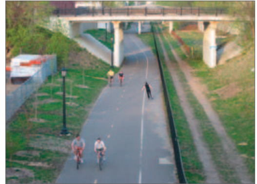
Above: The Midtown Greenway in Minneapolis has reserved enough land along its bicycle path to accommodate a transit line when funding becomes available.
