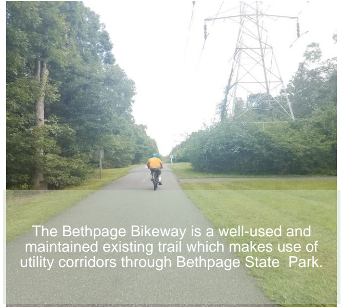
Some portions of the ROW in Nassau County are already unobstructed and accessible to adjacent residential properties for recreational purposes.
