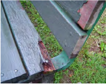
Bench was splintered and damaged
