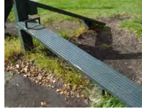
Missing loose-fill at exercise station
