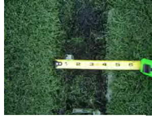
2 inch separation in turf
