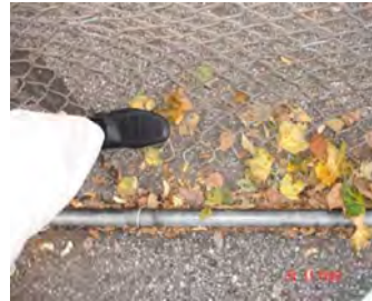
Missing tie-backs under basketball hoop
