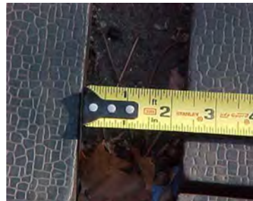
2 inch gap in safety surface
