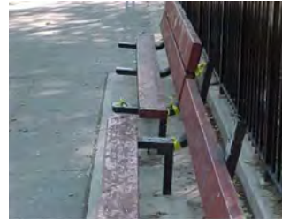
Benches missing slats
