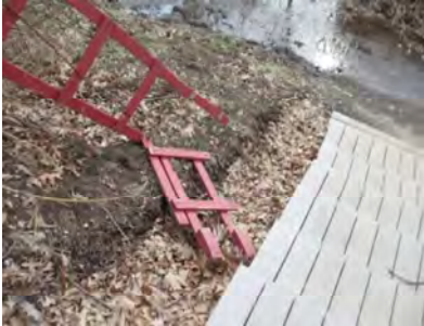
Damaged ice rescue ladder, Priority One Immediate Attention
