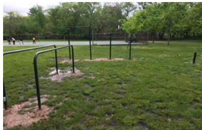
② POOR DRAINAGE
