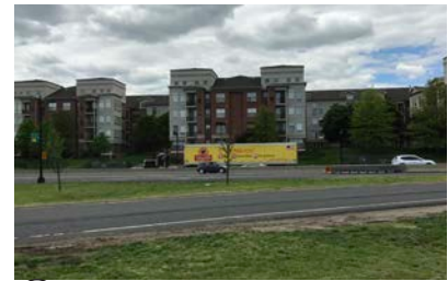
③ LACK OF GUARDRAIL ON 18
