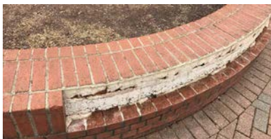
④ BRICKWORK NEAR ENTRANCE
