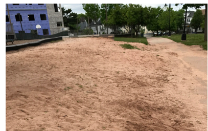
⑥ EROSION NEAR PLAYGROUND
