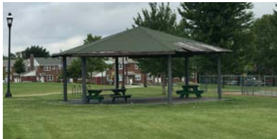
① DAMAGED PAVILION ROOF
