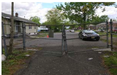
⑦ MAINTENANCE ENTRANCE
