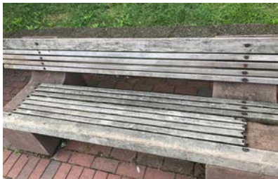
④ DAMAGED BENCH
