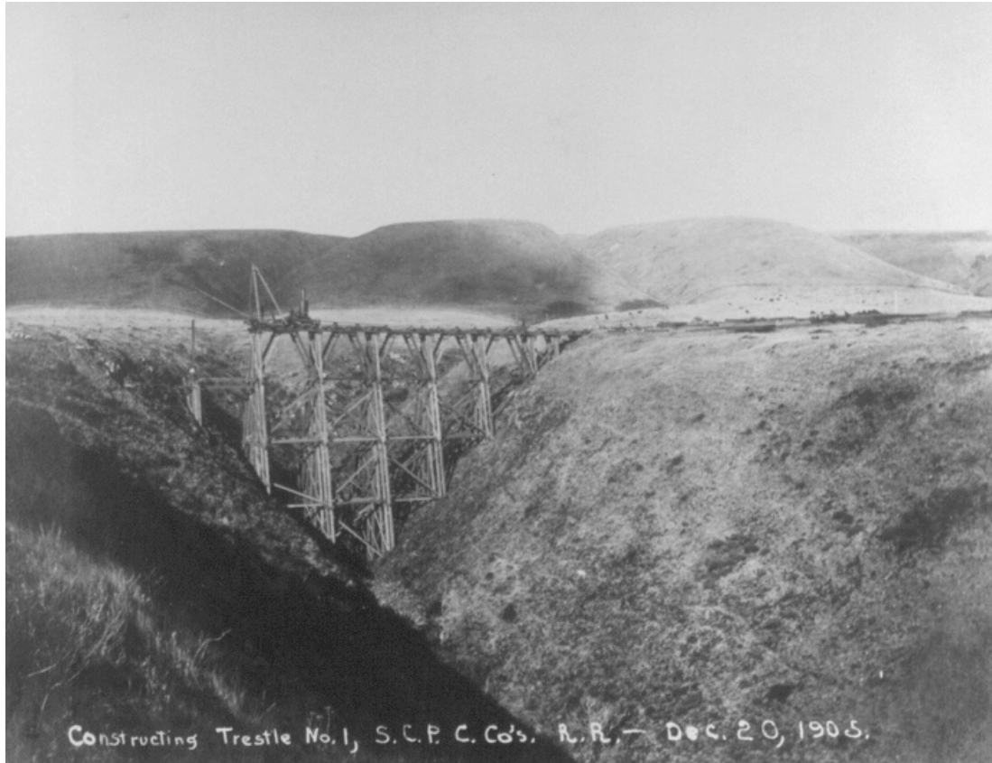
Photo 1-6: Construction of the Santa Cruz Portland Cement Company's Trestle No. 1, 1905
