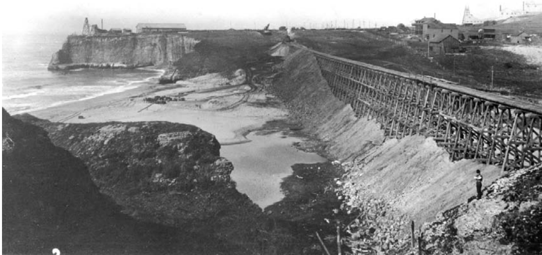
Photo 1-4: Filling the Trestle South of Davenport, View to the North to Davenport and the Cement Plant
